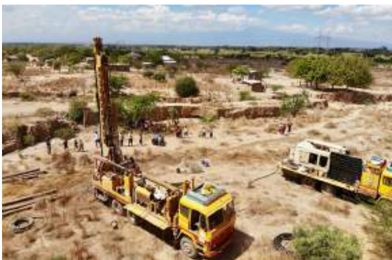
TATU Well · Drilling process, December 2018
